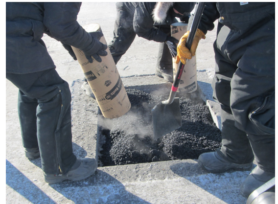
Above: Thanks to iHMA's induction heating method, asphalt repairs can now be made in any weather condition—including freezing or even sub-freezing temperatures.
